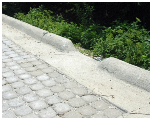
Figure 709-A: Cuts in the continuous curb allow for stormwater to be directed into landscaped areas.
